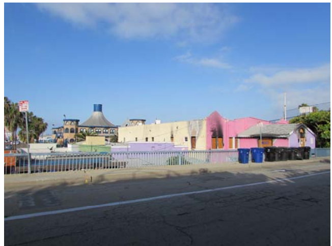
PHOTO - 4: East elevation context view, looking west
