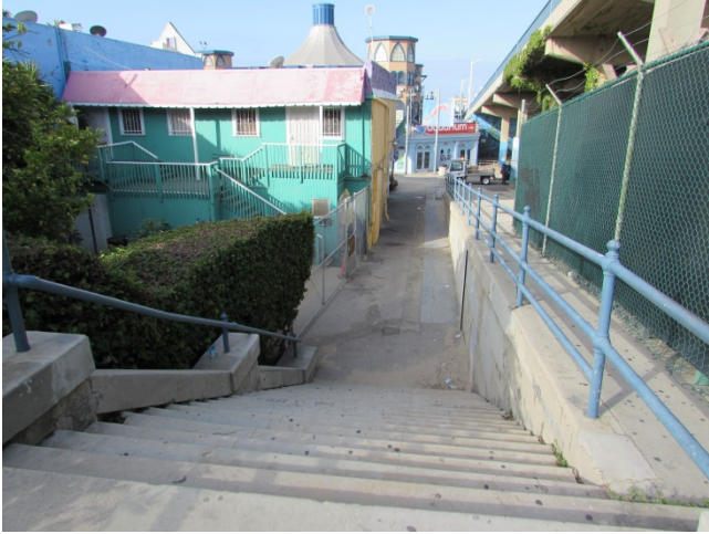
PHOTO - 13: Rear view, 1601 Ocean Front, looking west
