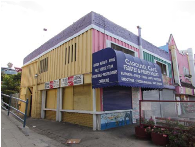
PHOTO - 7: 1601 Ocean Front Walk, looking southeast
