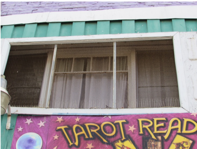
PHOTO - 15: Original tripartite detail at 1601 Ocean Front Walk
