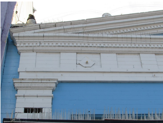
PHOTO - 17: Detail of cornice/parapet at 1611 Ocean Front Walk
