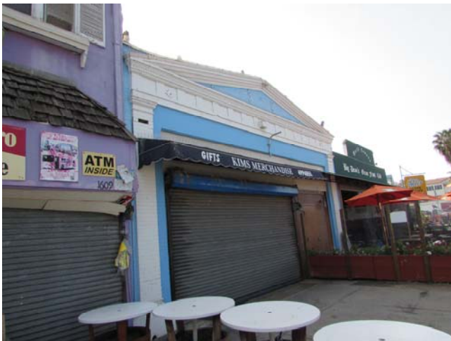
PHOTO - 9: 1611 Ocean Front Walk, looking southeast
