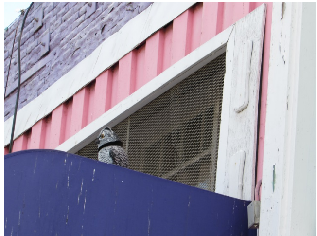
PHOTO - 16: Original tripartite detail at 1601 Ocean Front Walk
