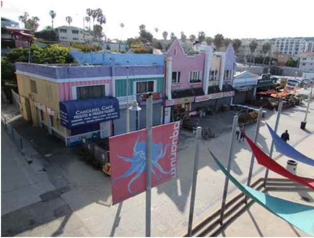
PHOTO - 1: Oblique, context view, looking southeast
